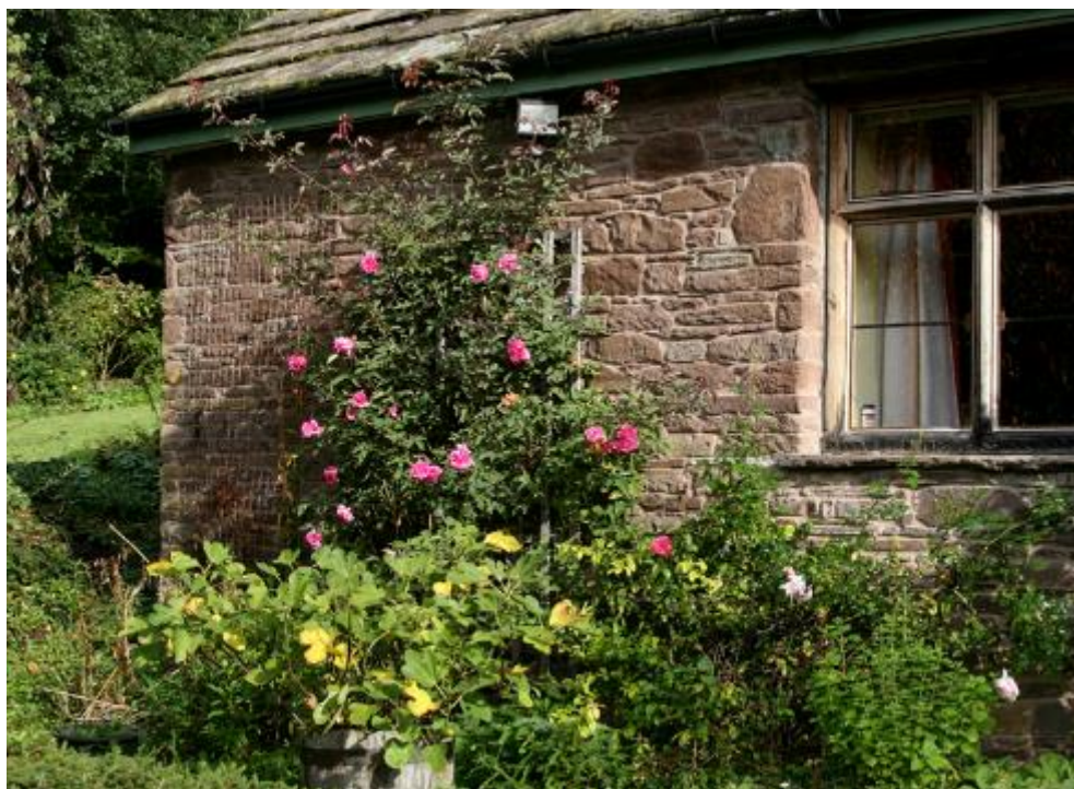
Local stone used to construct a new building in a rural setting (Liz Overstall)
